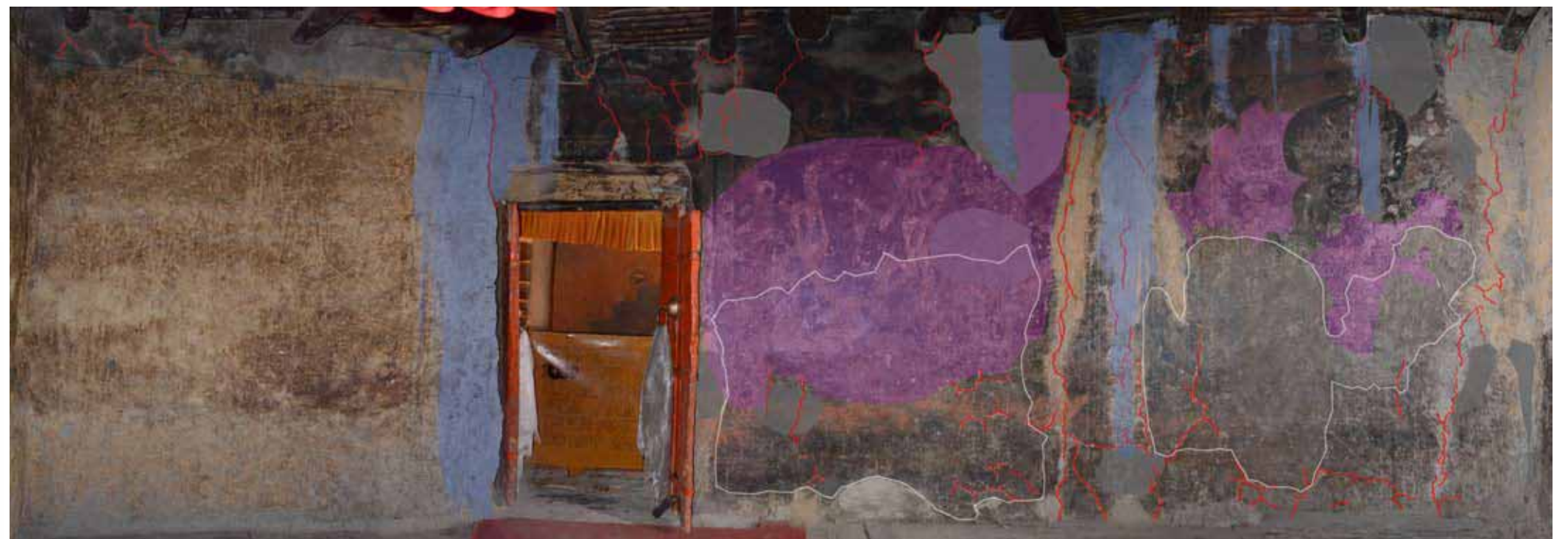
Map.6. The Dukhang East wall showing voids, cracks, washouts and drips, flaking and thinned painted surfaces
