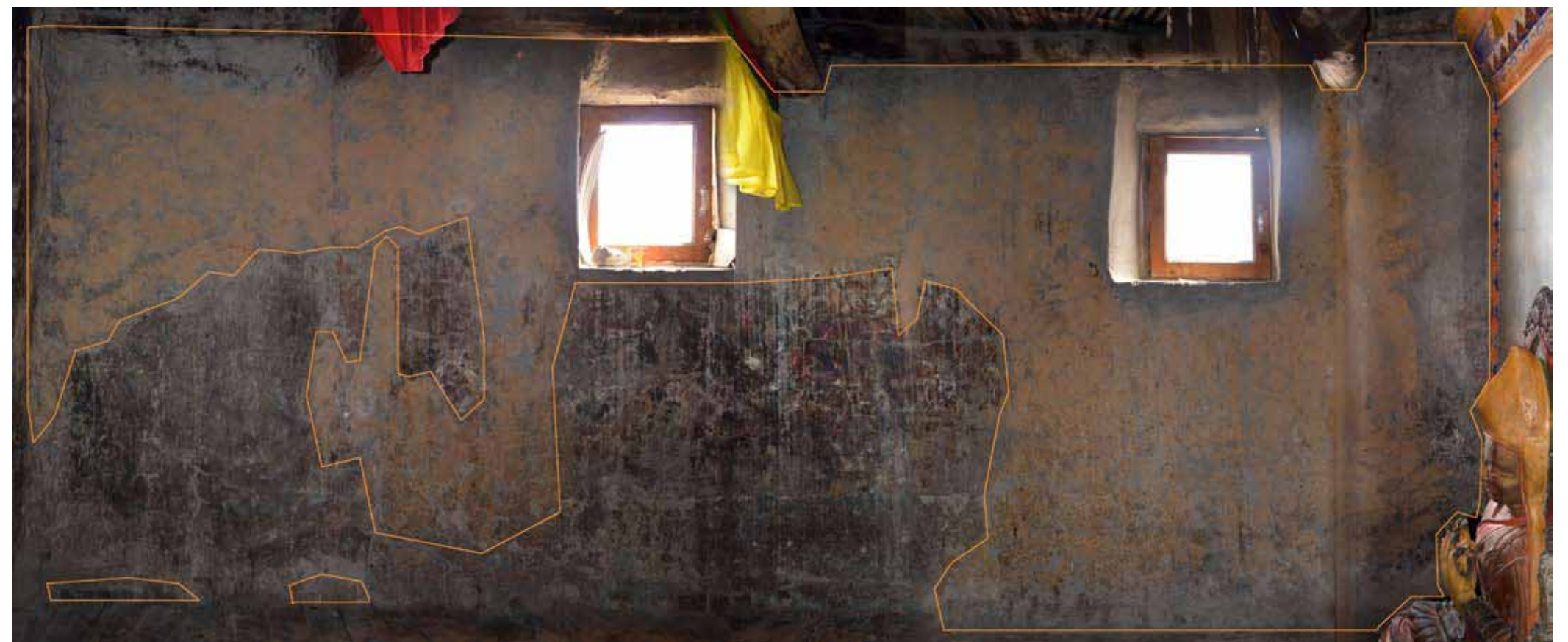
Map.8. The Dukhang South wall with the extent of undecorated plaster, repair and repainted surfaces indicated
