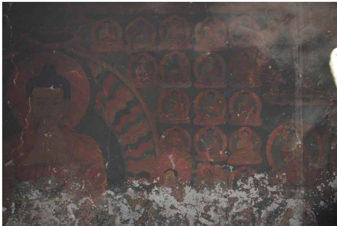
Fig.6. Wall behind the wooden construction with intact although decayed wall paintings
