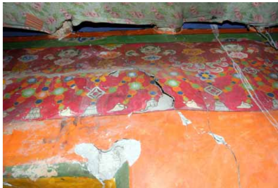
Fig.2. Voids, cracks and losses of paint layer and plastering
