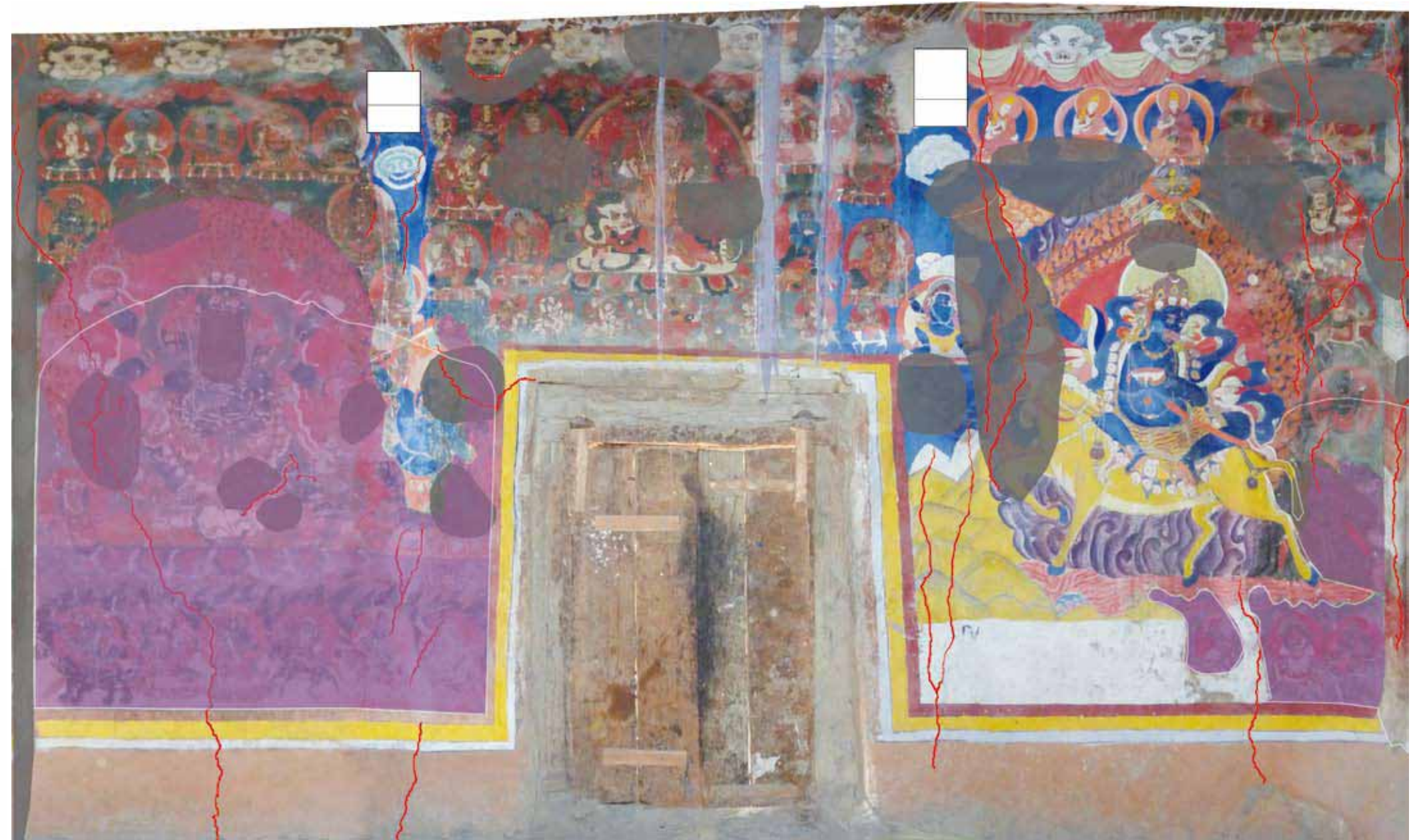
Map.12. The Lhakhang Gongma Northeast wall showing voids, cracks, washouts and drips, flaking and thinned painted surfaces
