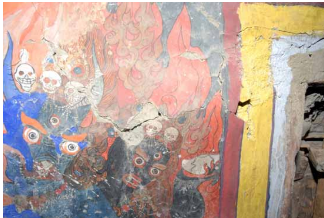
Fig.11. Voids, cracks and losses
