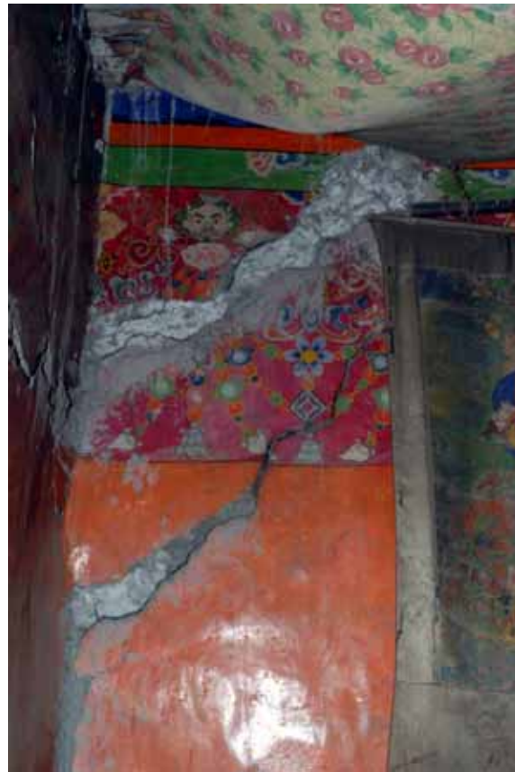
Fig.1. Deep cracks and losses of paint layer and plastering
