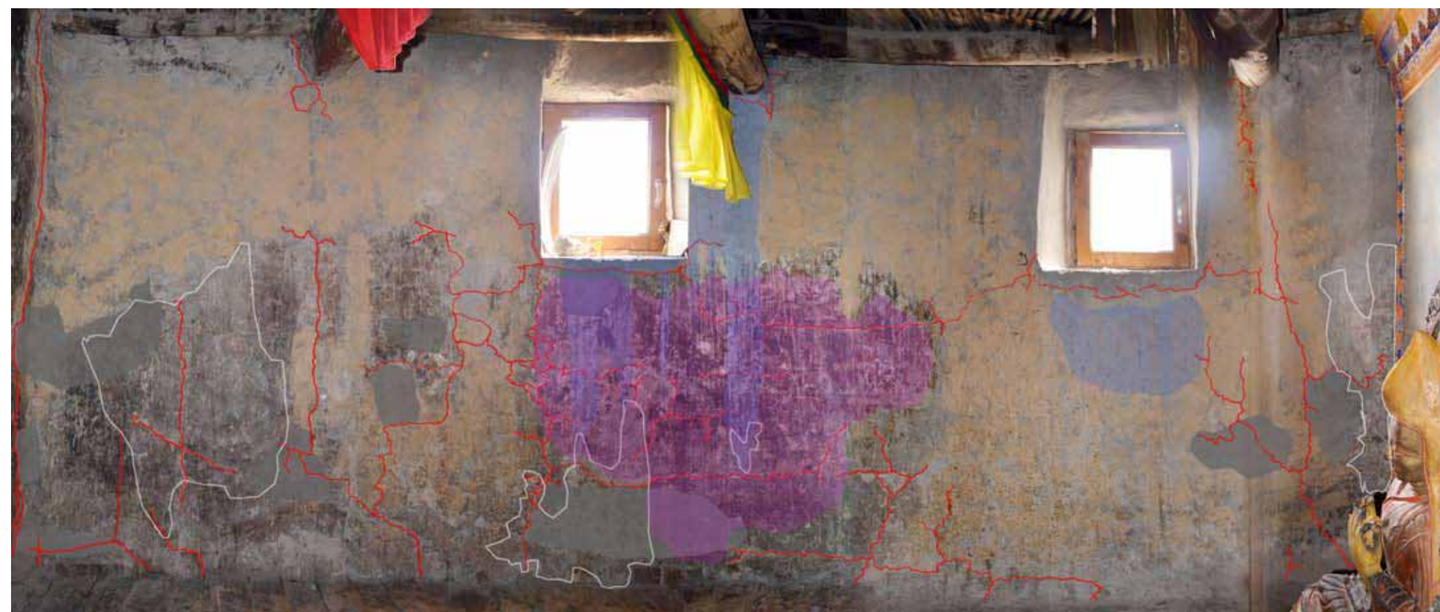
Map.9. The Dukhang South wall showing voids, cracks, wahouts and drips, flaking and thinned painted surfaces
