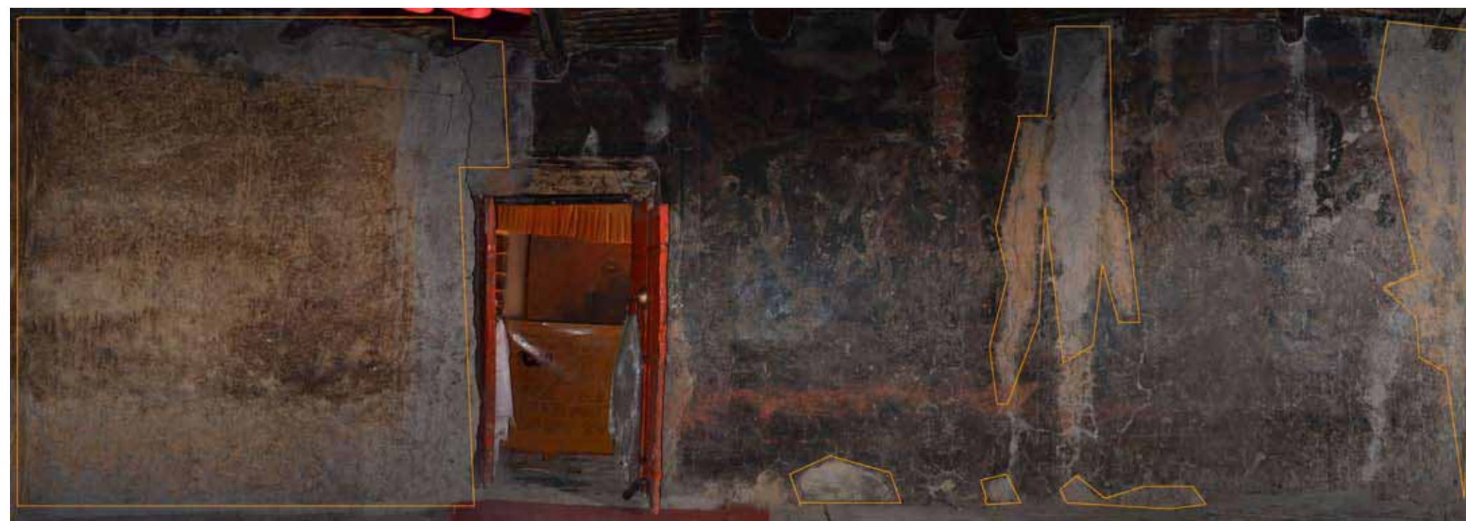
Map.5. The Dukhang East wall with the extent of undecorated plaster, repair and repainted surfaces indicated
