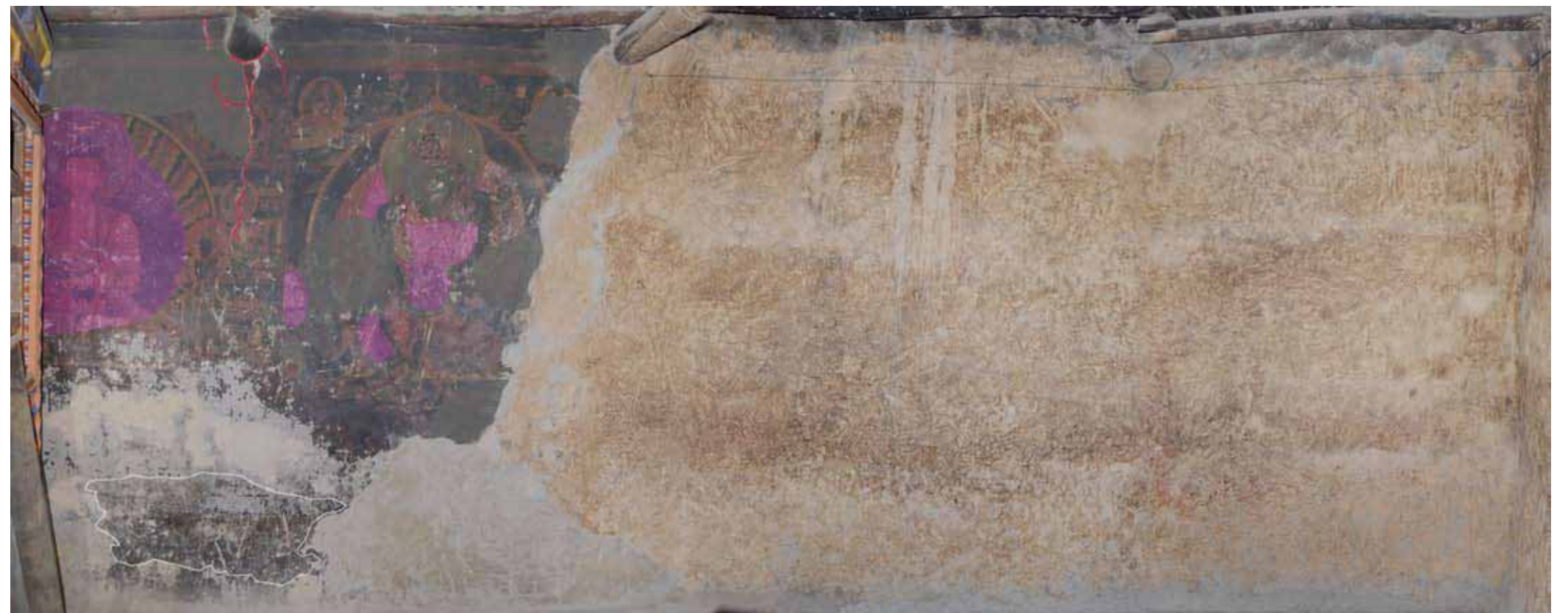
Map.3. The Dukhang North wall showing voids, cracks, flaking and thinned painted surfaces
