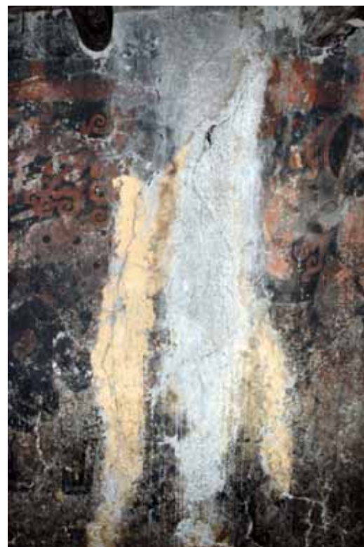
Fig.12. Repair-filling, deposits in form of channels
