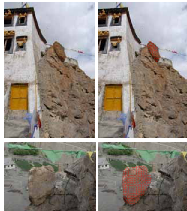
Figure 3.24 Potentially unstable rock block adjacent to northern side of Tower.
