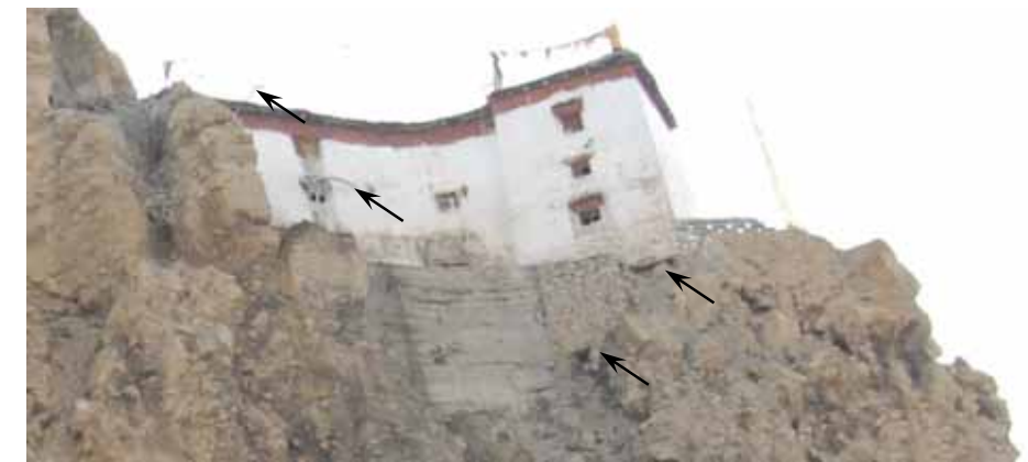
Figure 3.18 Southern side of Ancient Monastery, showing area of prior remedial cliff work (note two drainage pipes, partial undermining at of building foundation at right corner, and partial undermining of block/mortar slope repair).
