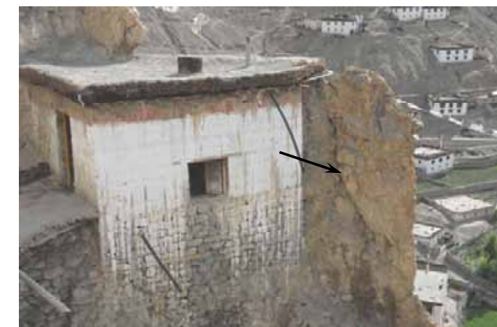
Figure 3.8 Tensile fracturing of the Dangkhar Bimrock.
