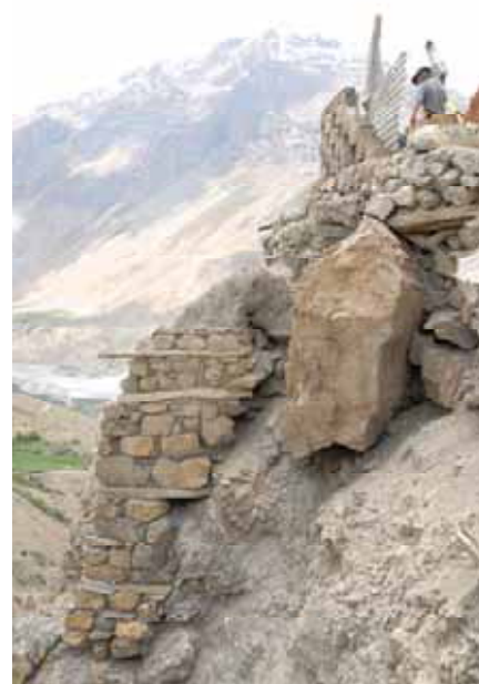
Figure 3.17 Partially undermined large block along eastern side of Ancient Monastery.
