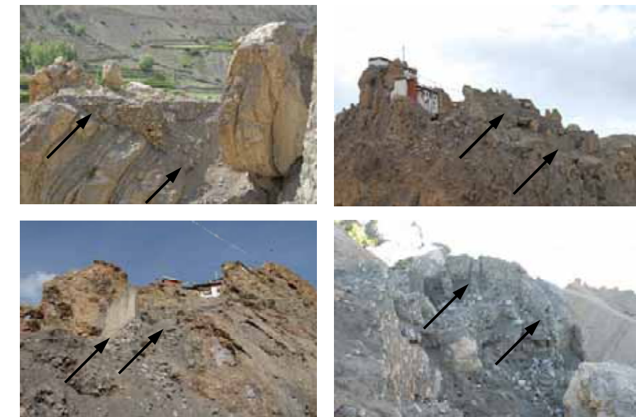
Figure 1.5 Foundation remnants within Areas 1 and 2 of Figure 1.4 (arrows point to the foundation - earth interface).
