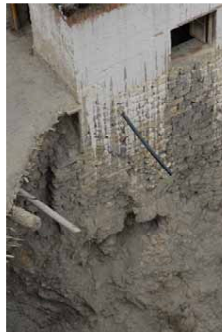
Figure 3.21 Detail of undermined Kitchen foundation.
