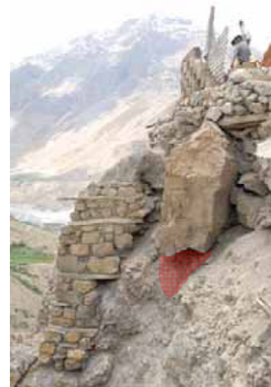
Figure 4.5 Underpin large block along eastern side of Ancient Monastery.
