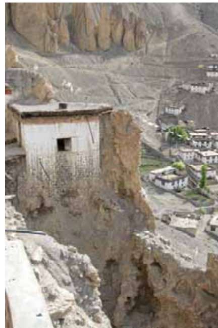
Figure 3.16 Erosion gully along eastern side of Ancient Monastery, view to north (note four drain pipes discharging to gully)
