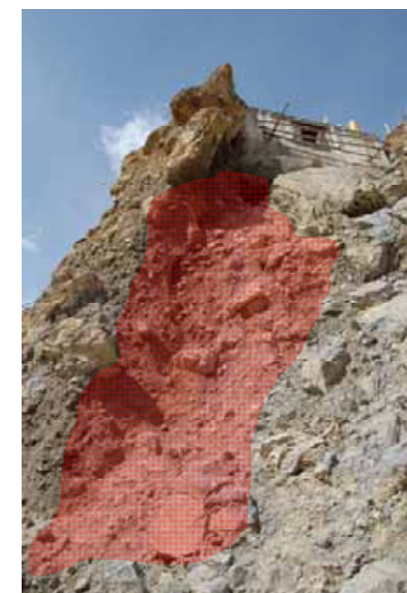
Figure 4.8 Shotcrete protection and underpinning along northern side of Museum.
