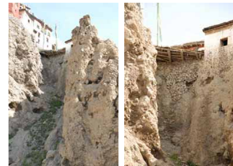
Figure 3.15 Erosion gully along eastern side of Ancient Monastery and southern side of Kitchen (note partial undermining of block-mortar work in the erosion headwall).
