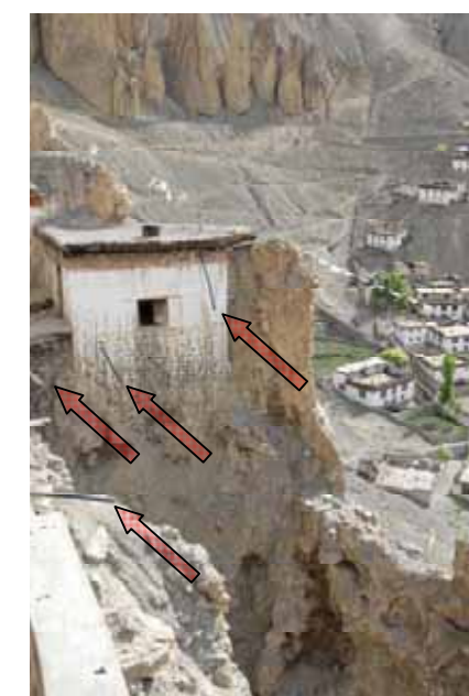
Figure 4.4 Prevent water discharge into gully along eastern side of Ancient Monastery.
