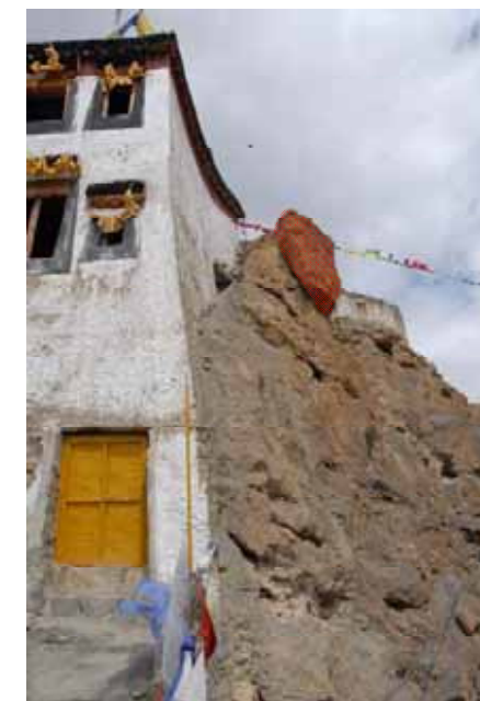
Figure 4.11 Potentially unstable block along northern side of Tower.
