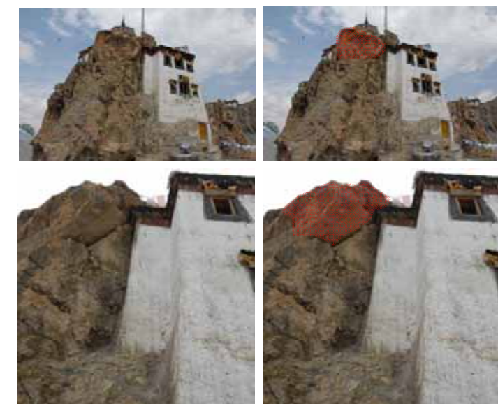
Figure 3.23 Potentially unstable rock block bordering southern side of Tower
