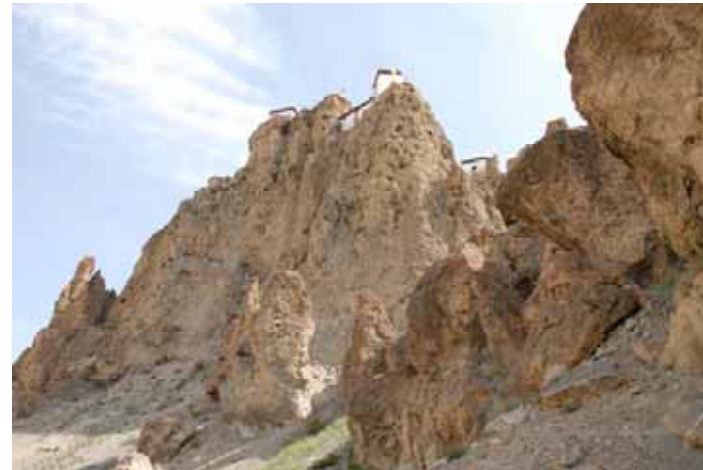
Figure 2.12 Bimrock foundation of the Ancient Monastery Complex.
