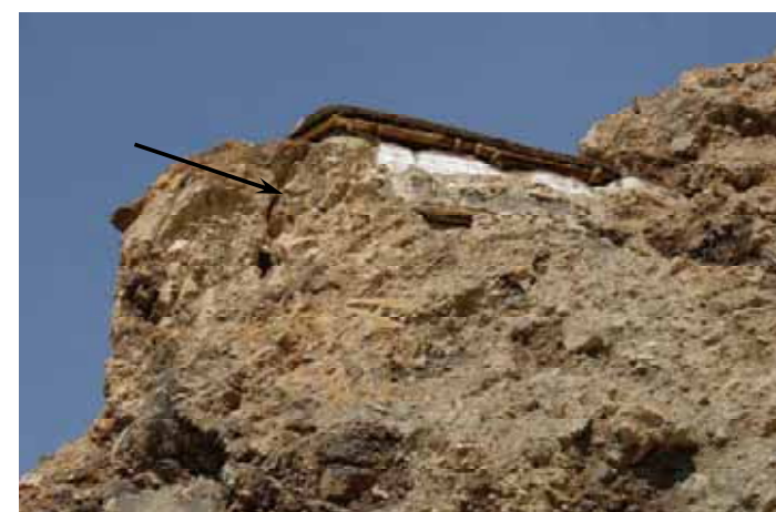
Figure 3.9 Tensile fracturing adjacent to monastery structures.
