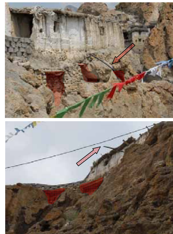
Figure 4.13 Underpin foundation elements along eastern side of Upper Temple, and prevent water discharge over cliff.
