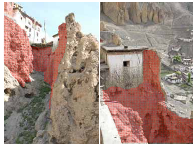
Figure 4.2 Shotcrete protection along eastern side of Ancient Monastery and southern side of Kitchen.
