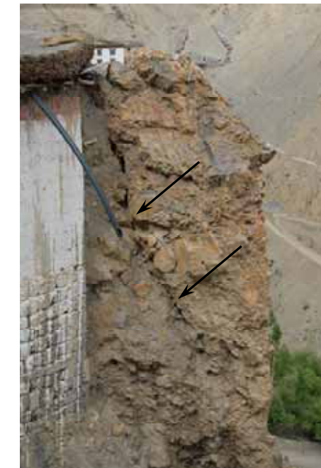
Figure 3.22 Tensile fracturing of bimrock fin along eastern side of Kitchen.
