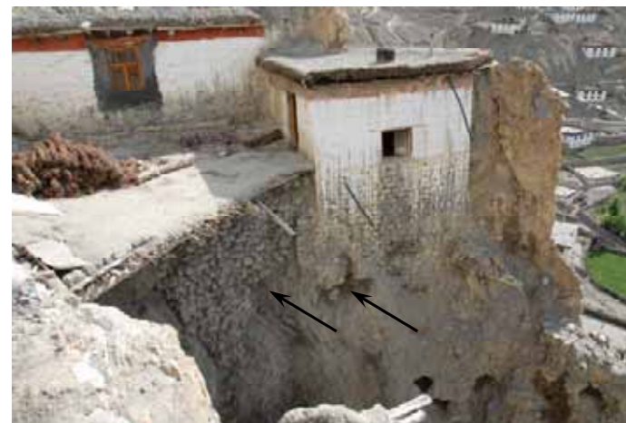
Figure 3.20 Partial undermining of block/mortar slope repair and foundation along southern side of Kitchen (note drain pipes).
