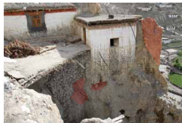
Figure 4.9 Underpin foundation elements along southern side of Kitchen.
