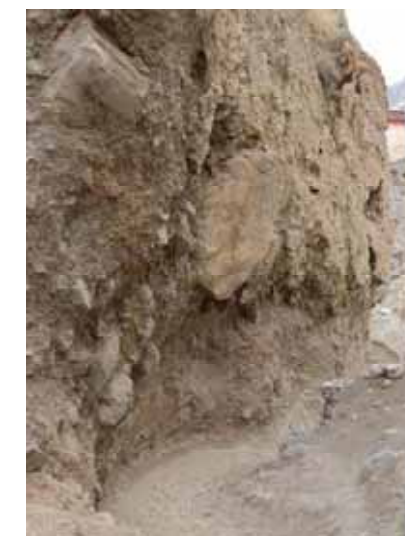
Figure 3.12 Differential erosion of block and matrix components, leading to the undermining and loosening of large block components
