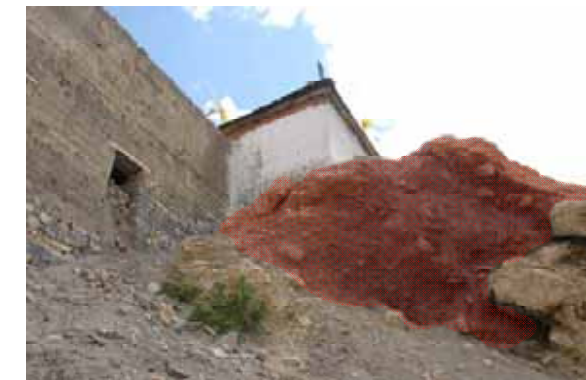
Figure 4.14 Overhanging slope at Castle of the Nono.
