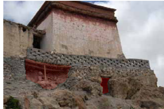
Figure 4.12 Underpin foundation elements along western side of Upper Temple.
