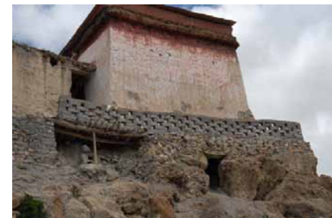
Figure 3.27 Foundation undermining along western side of Upper Temple (note wood post and beams).
