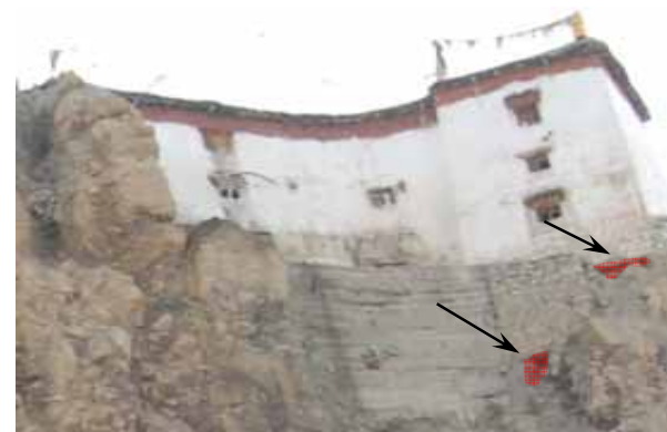
Figure 4.6 Underpin foundation elements along southern side of Ancient Monastery.
