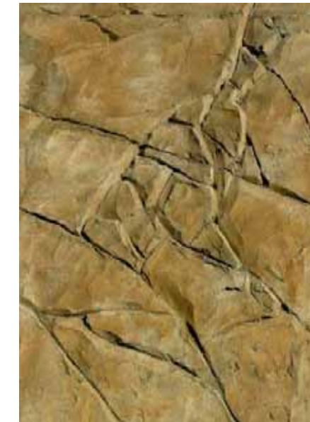
Figure 4.3 Example of textured and pigmented shotcrete wall.
