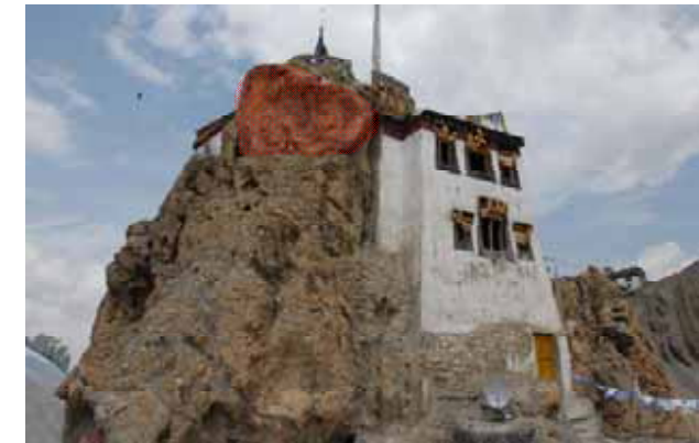
Figure 4.10 Support potentially unstable block along southern side of Tower.
