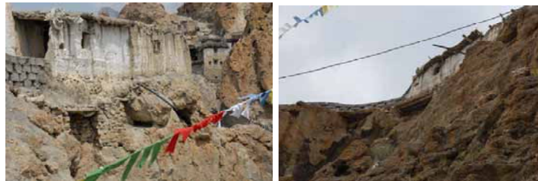
Figure 3.28 Foundation undermining along eastern side of Upper Temple (note block and mortar underpinning, spanning timber beams, and drainage pipe).
