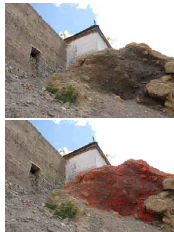
Figure 3.29 Castle of the Nono, depicting overhanging bimrock outcrop along eastern side of structure.
