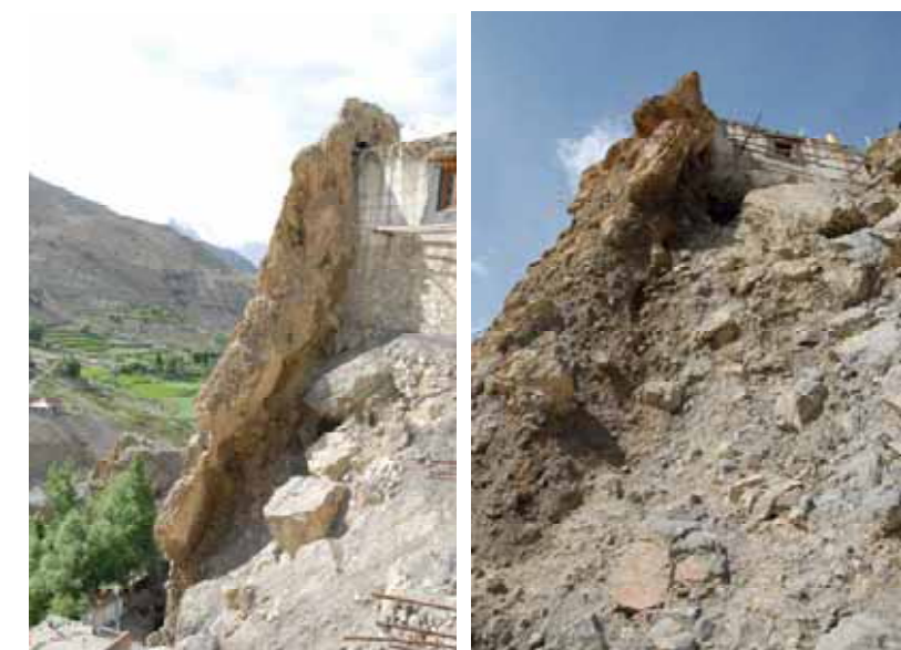
Figure 3.19 Erosion rill and partial undermining of foundation along northern side of Museum (note bimrock fin along eastern side).
